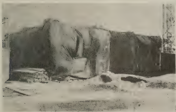
FRESHLY PLACED CONCRETE PROTECTED BY CANVAS
